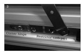
Fix the frame part of the restrictor at the cill as on shown the picture.
